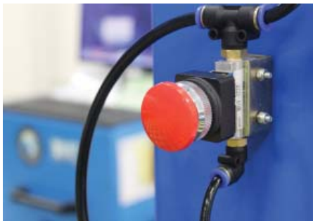
Air Lock Release Valve
